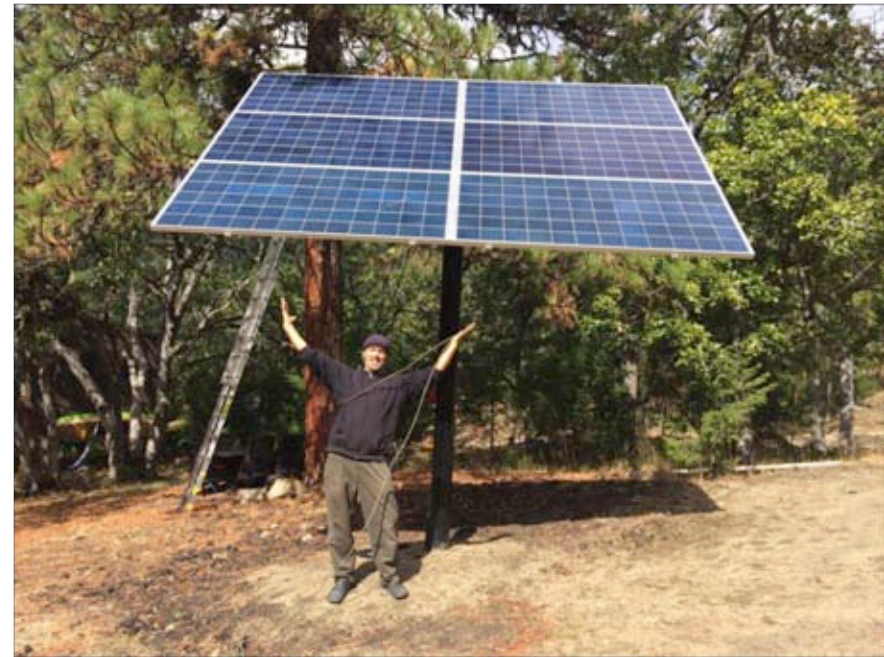
“Tiny House Build” solar array!
